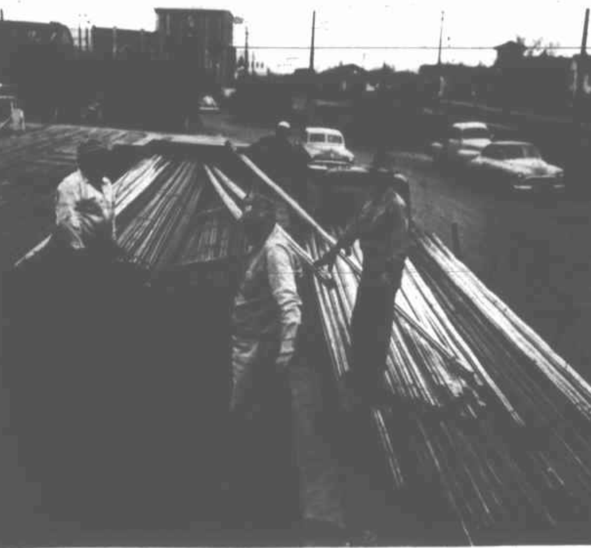
Louis Kohleffel, center, owner of Eagle Lake Pipe Company, is shown with his first trainload of over 1000 pipe from Belgium. Shipment in 1972 through 1973.
